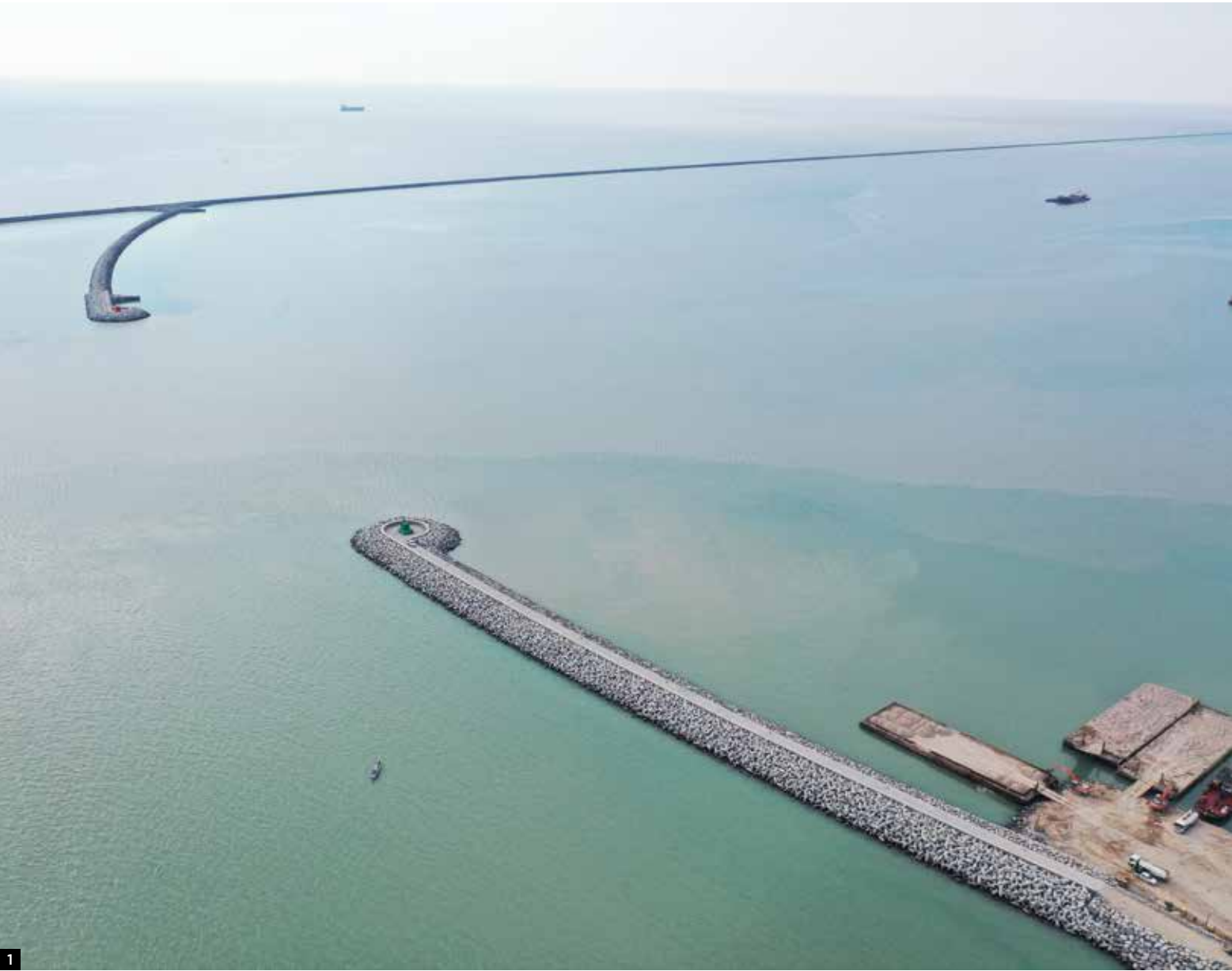
1 AL-FAW BREAKWATER, IRAQ - Construction of a 15.952 Kilometer-long riprap breakwater - Ranked as the Longest Breakwater in the world by Guinness on April 2nd, 2020 - Officially registered as Guinness World Record
