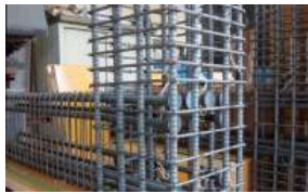
Threaded rebar construction
