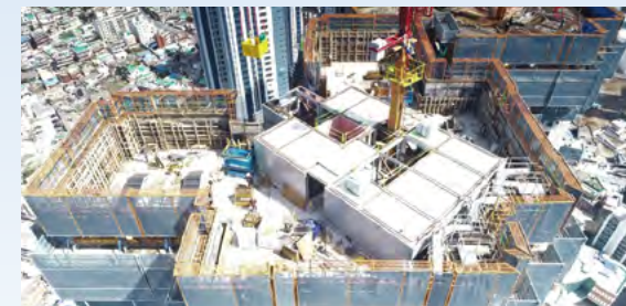
▲ Rooftop steel frame modular construction(Haeundae Central)
