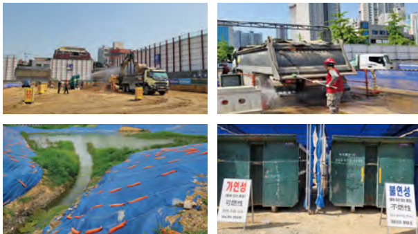
▲ Spraying and washing the wheels in loading, sediment basin, and separate storage of waste(from upper left)
